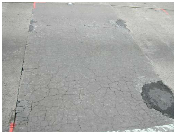
Figure 3. Cracking in full-depth repair (TxDOT, 2011)
